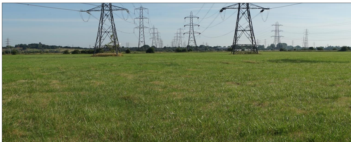
Figure 1.1: Main development site baseline photograph – looking north from Tilbury Substation.
