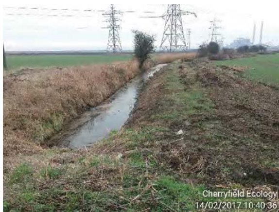
Figure 8: Example of ditch system, cleared to the left.
