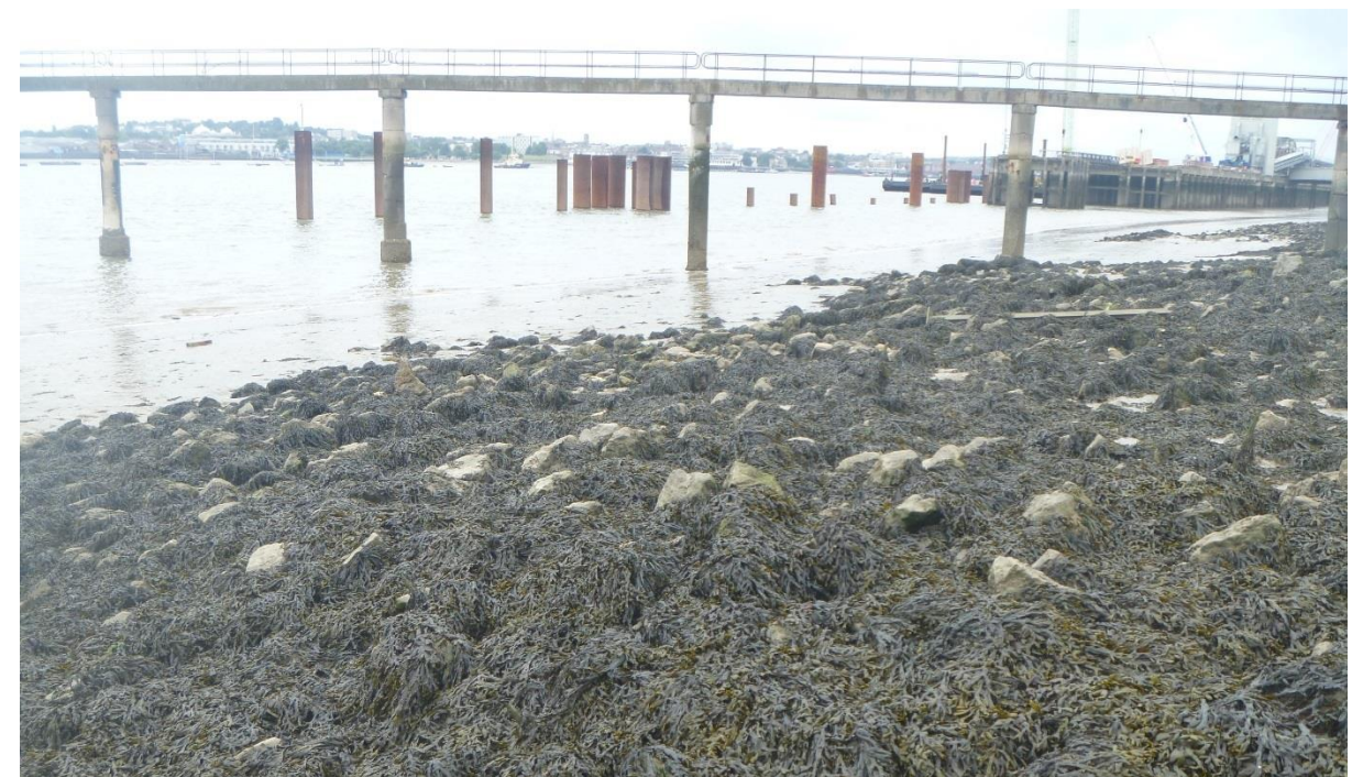
Figure 3.3: Tilbury2 RoRo pontoon under construction at the time of writing.
