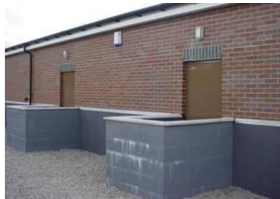
Figure 6.4: Exterior of building displaying flood protection and bunding to access and emergency exit doors (ENA ETR138 Annex 1)
