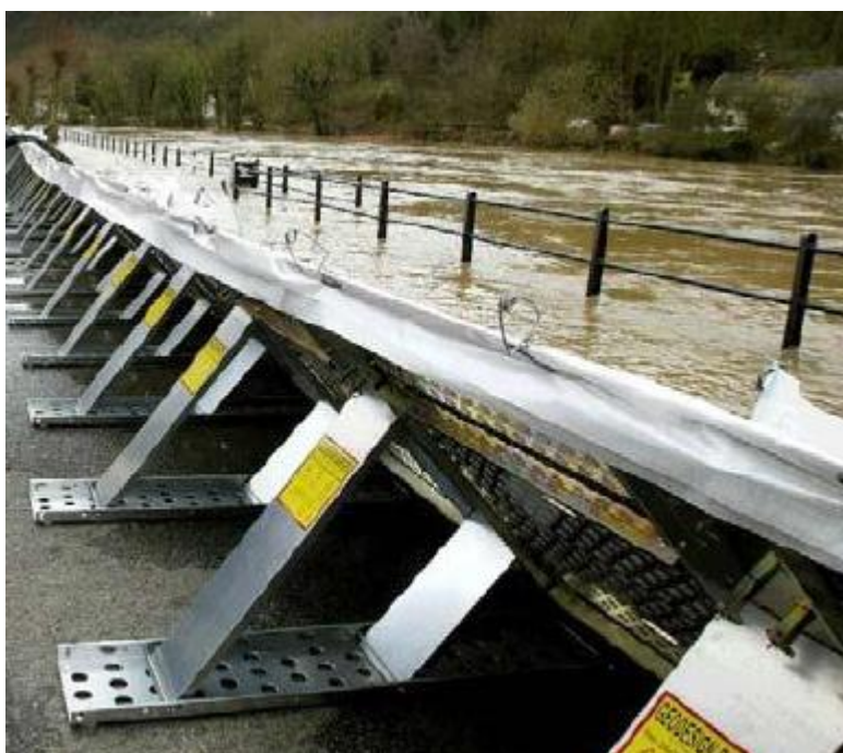
Figure 6.10: Temporary flood defence system (ENA ETR138 Annex 1)
